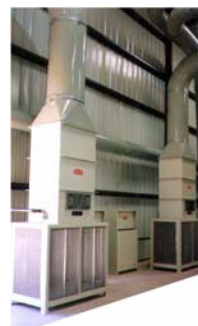
Samuel Jackson heaters are designed and built specifically for pull-through drying.
