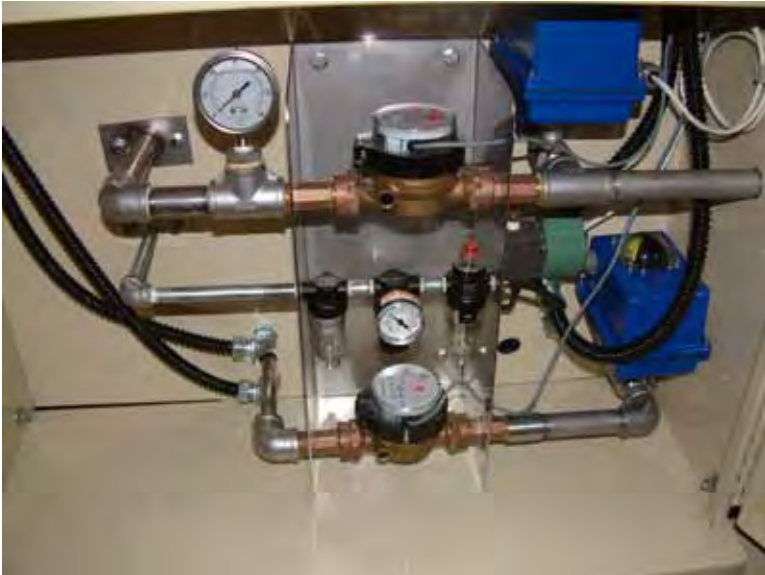
Water Watch meters are housed in the lower cabinet and help measure the ROI of moisture restoration at your gin.
